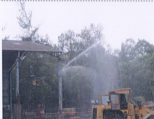
Sprinkler systems are in place to mitigate the Fugitive emissions – Coal and ash handling area
