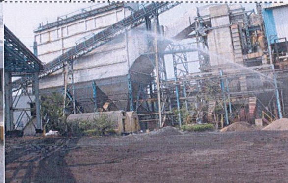
Sprinklers in fuel handling area
