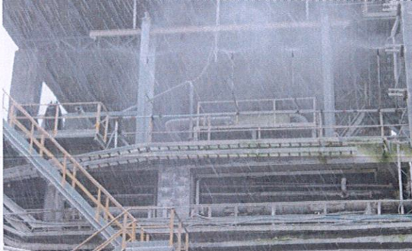
Sprinkler systems – Limekiln area
