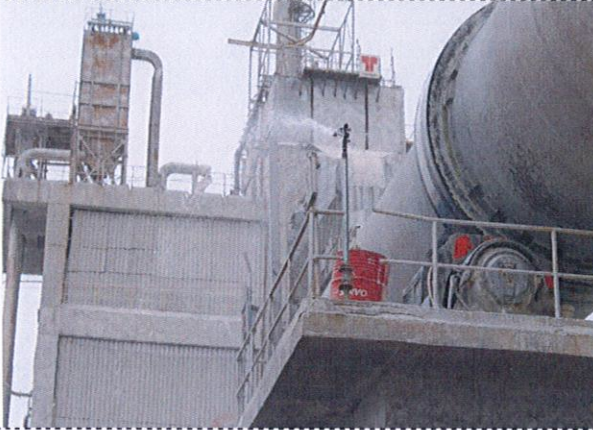
Sprinkler systems – Limekiln area
